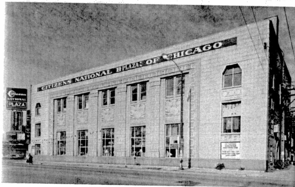
Chicago terra-cotta manufacturers embraced avant-garde Art Deco-style ornamentation in the late 1920s. Top: Northwestern Terra Cotta Company modelers at work. Bottom: The Laramie State Bank Building (a designated Chicago Landmark at 5200 W. Chicago Ave.) is a fine example of polychromatic terra cotta, popular in the late 1920s.
